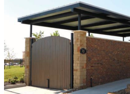
Example of screened dumpsters
