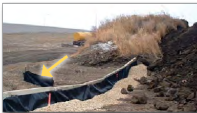
Figure 17. Back of silt fence on part of the stock pile's perimeter
