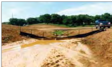
Figure 8. Proper installation, bottom of both ends are above the top of the middle
