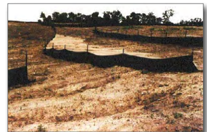
Figure 2. Create manageable sediment storage areas
