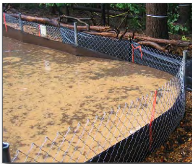
Figure 11. Chain link supported silt fence
