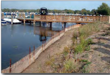
Figure 21. Silt fence protecting a lake shore
