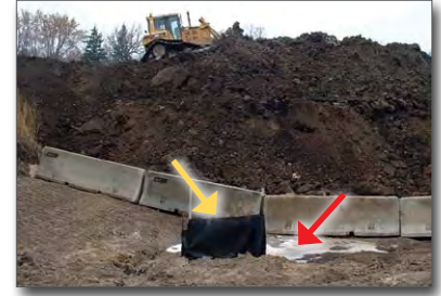
Figure 18. Front of silt fence on part of stock pile's perimeter
