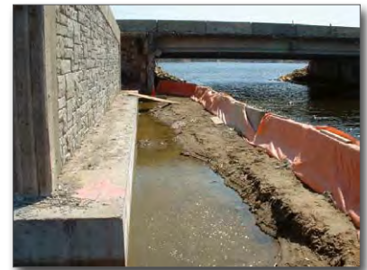
Figure 19. Silt fence for bridge abutment excavation
