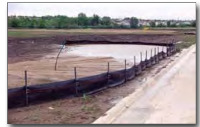
Figure 10. Gentle slopes may require a silt fence
