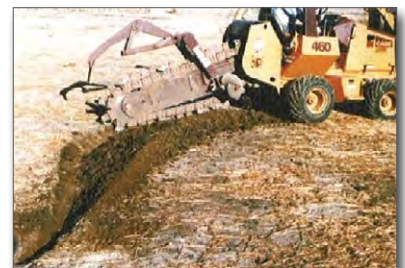
Figure 15. Trenchers make a wider excavation at turns
