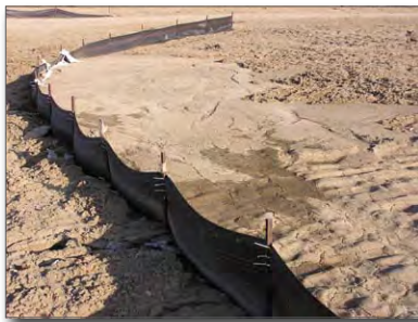
Figure 1. Silt fence retaining sediment
