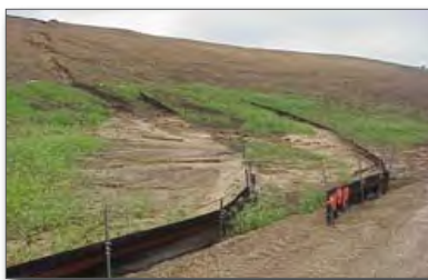
Figure 23. New silt fence below the old fence
