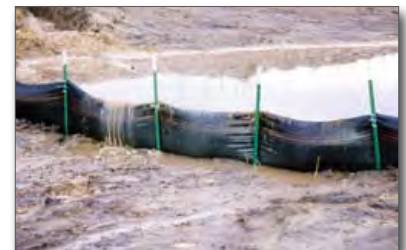
Figure 3. Water should not flow over the filter fabric during a normal rainfall
