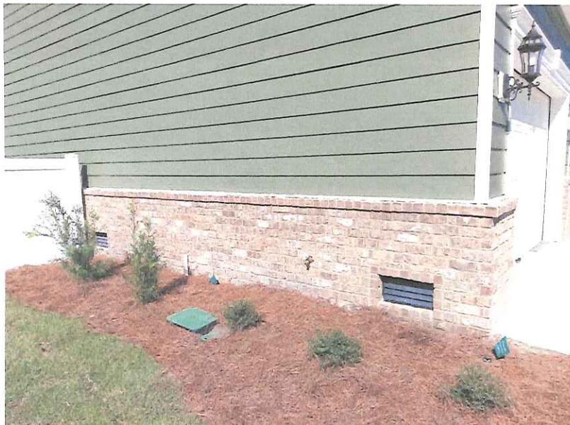
Left Side View taken 10/23/2017 showing Engineered Flood Vents
