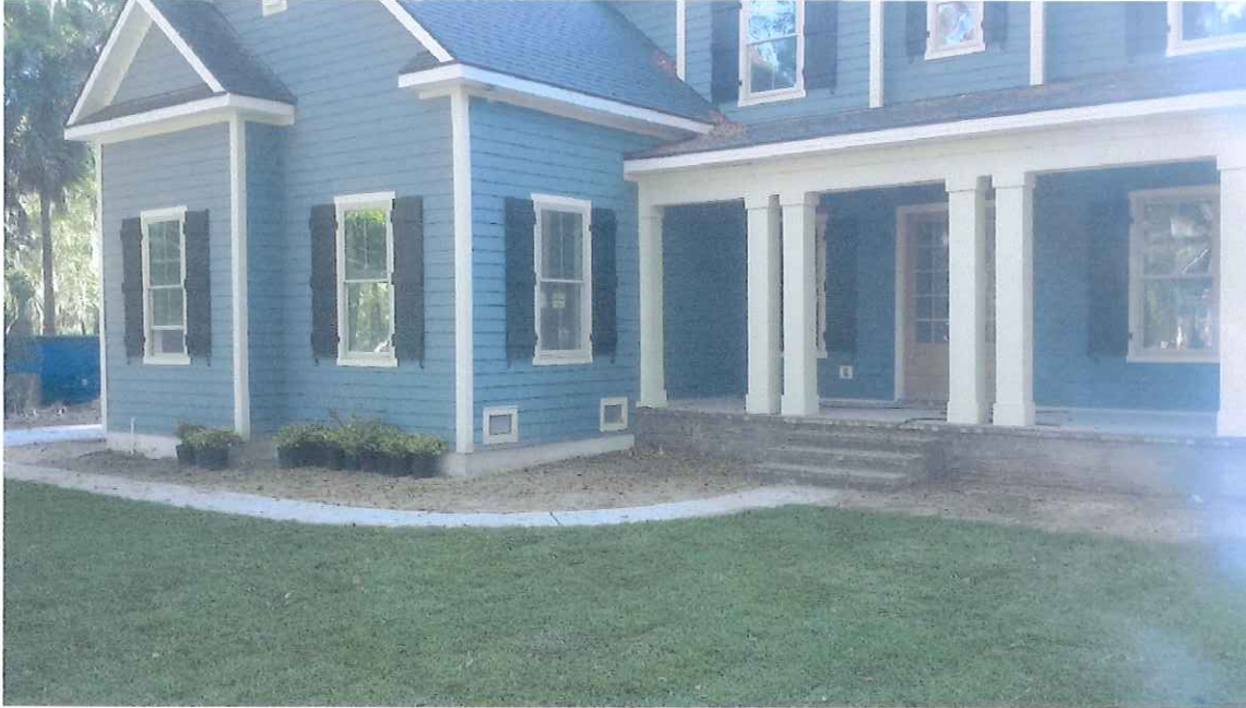
Front Right of Garage showing Smart Vents
