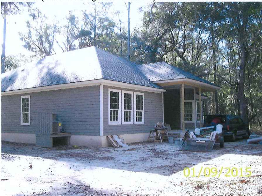
Rear View (with A/C on right side of house)
