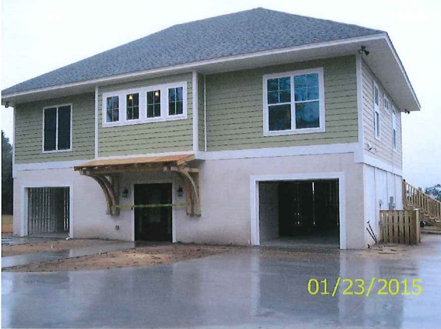
Front View and Right Side View (showing lowest servicing equipment C2e, An A/C unit, located behind wood fencing)
