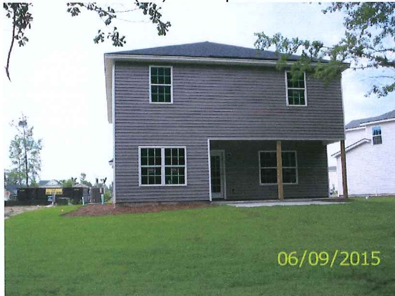
Rear View – A/C unit (C2e) on left in photo.
