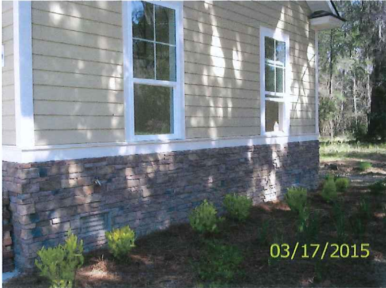
Front of garage showing typical Smart Vents
