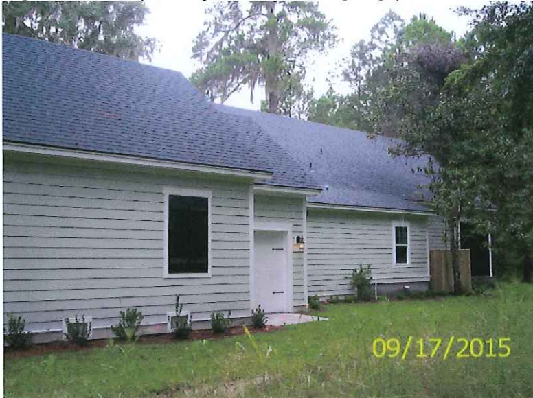
Right Side View (showing Smart Vents in garage)
