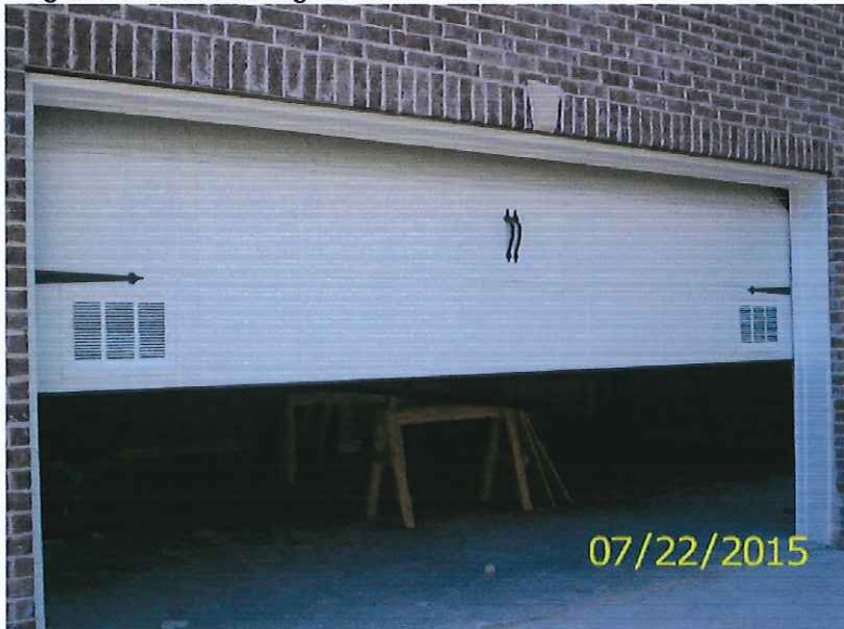
Regular Vents in Garage Door
