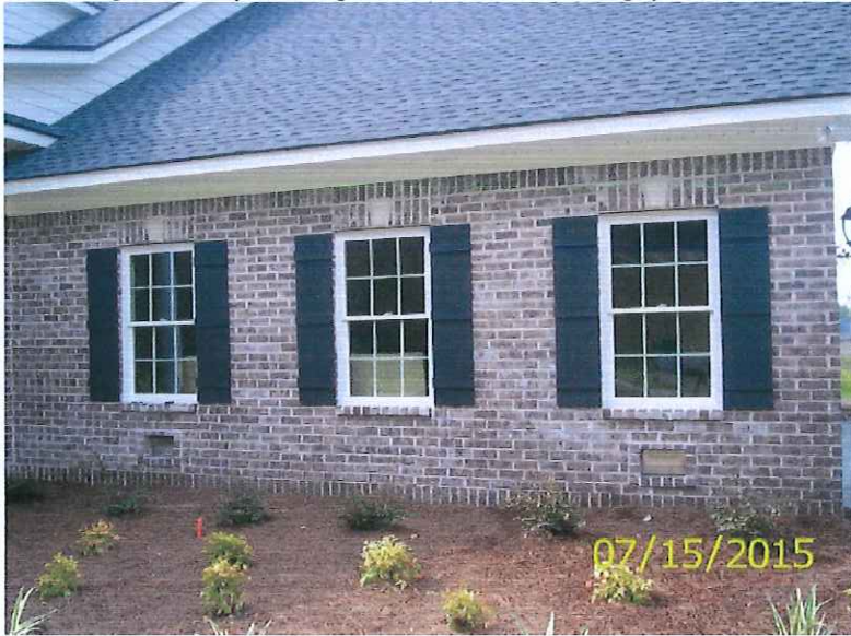
Front Right View (Showing Smart Vents in Garage)
