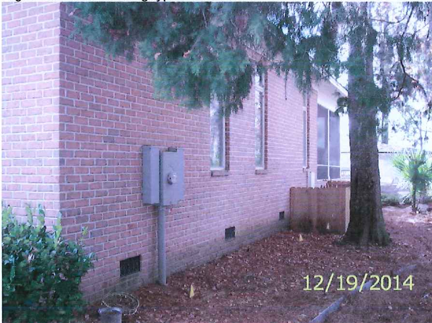
Right Side View showing typical flood vents
