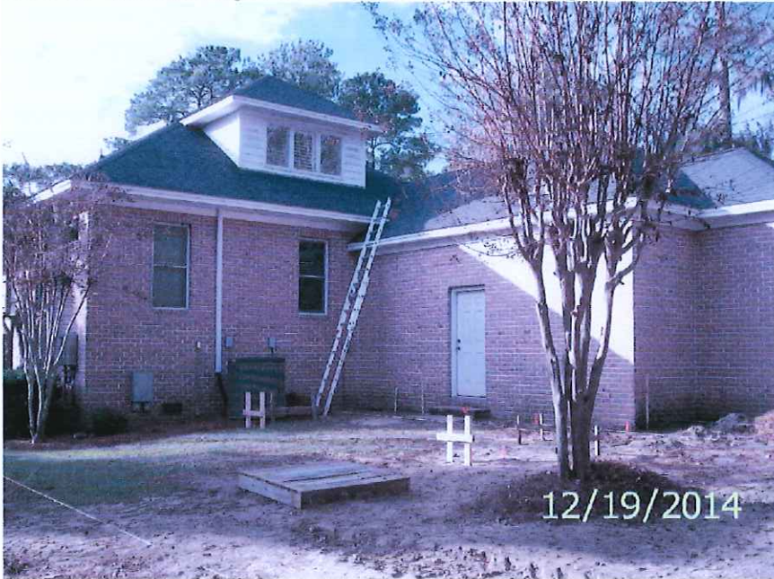
Left rear View showing A/C and rear of attached garage
