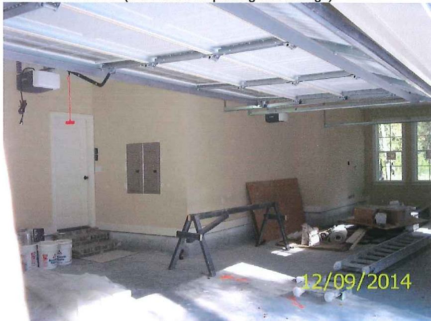
Inside enclosure A8 (to be used for parking and storage)
