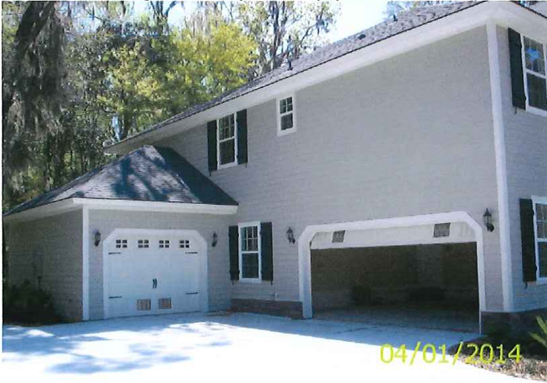
Left Side View showing garage #1 (opened door) and garage #2 There exists 4 regular vents per door (2 painted and 2 unpainted).
