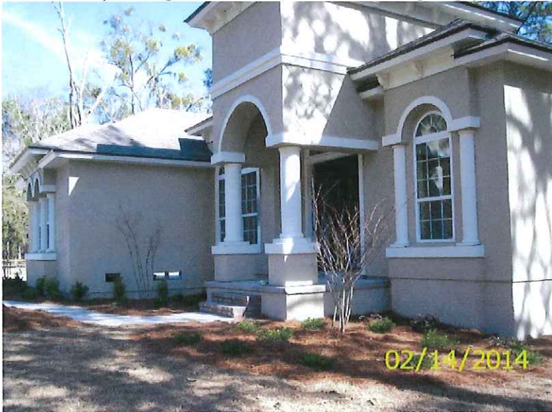
Front View (showing Smart Vents in back side of garage)
