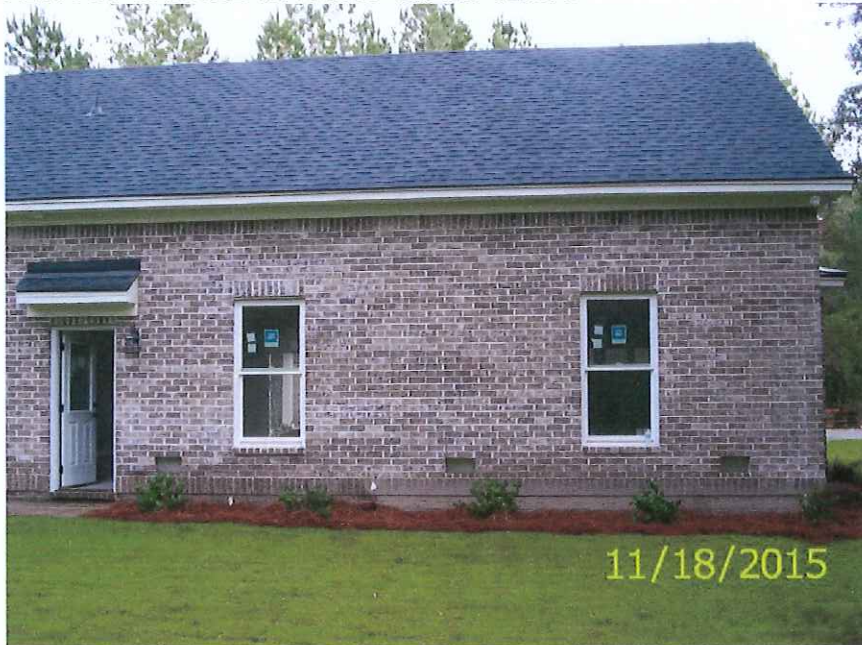
REAR OF GARAGE SHOWING SMART VENTS
