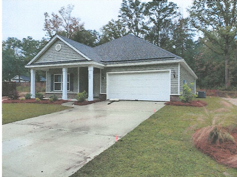
Front View taken 11/15/2019 showing the lowest servicing equipment for C2e
