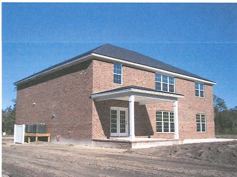
Right Side View taken 11/21/2019 showing lowest servicing equipment for C2e
