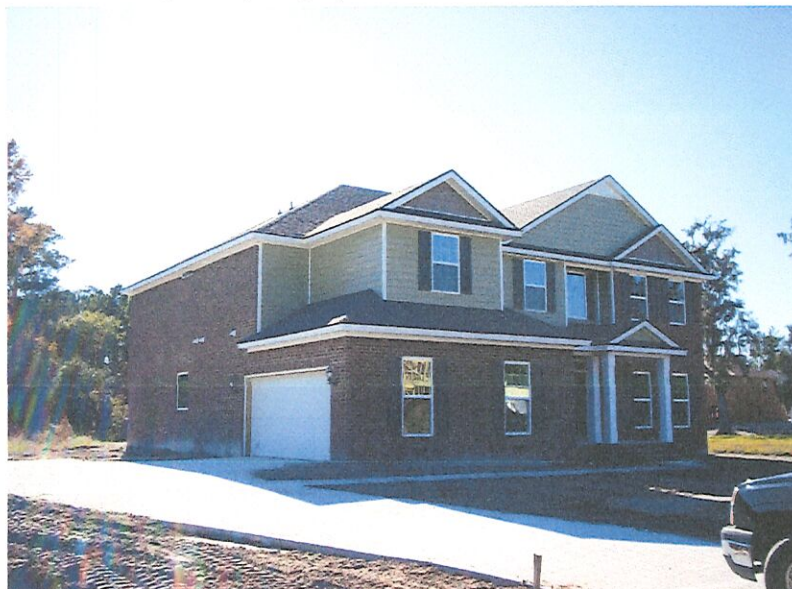
Front View taken 11/21/2019 showing flood vents in front and in garage door
