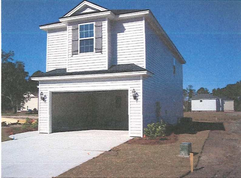
Front View taken 12/04/2019 showing the lowest servicing equipment for C2e (at right in photo)
