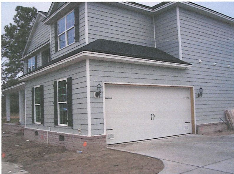
Front Right View taken 01/31/2020 showing engineered and regular flood vents
