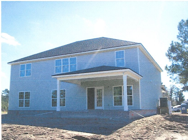
Rear and Left Side View taken 01/28/2020 showing the lowest servicing equipment for C2e
